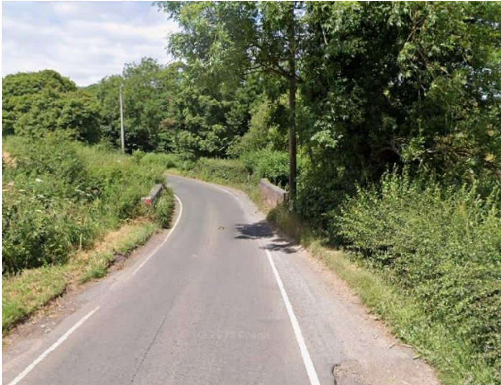
Plate 3-1: Single Lane Carriageway Over Existing Bridge in Norton
