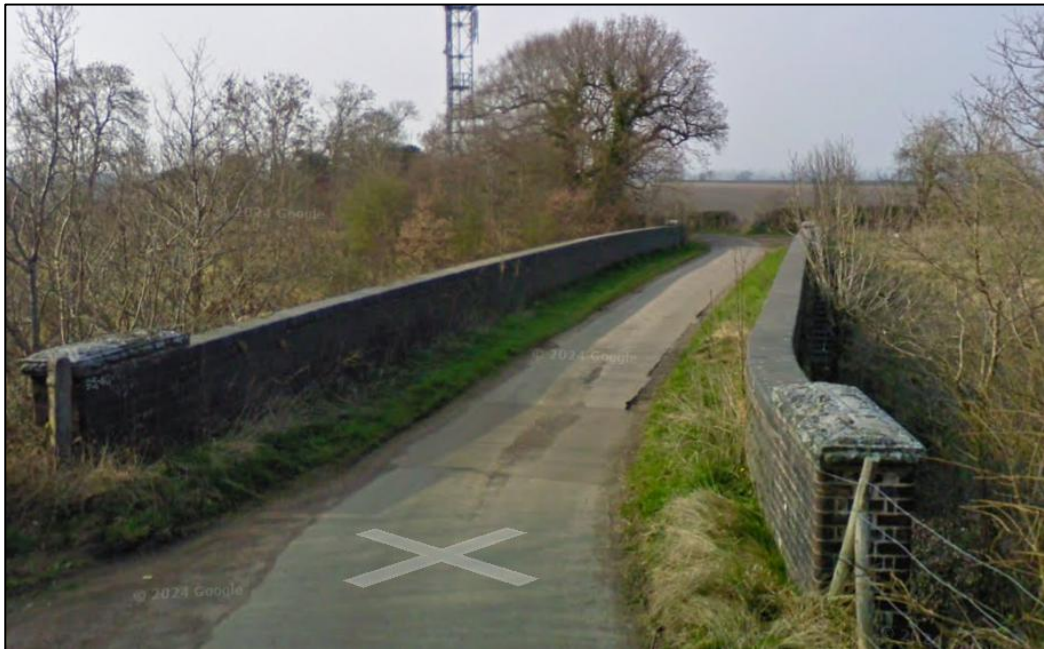
Plate 3-8: Narrow Railway Bridge between Hullavington and Farleaze
